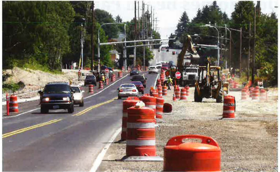
Reducing long delays by shifting traffic to temporary lanes
